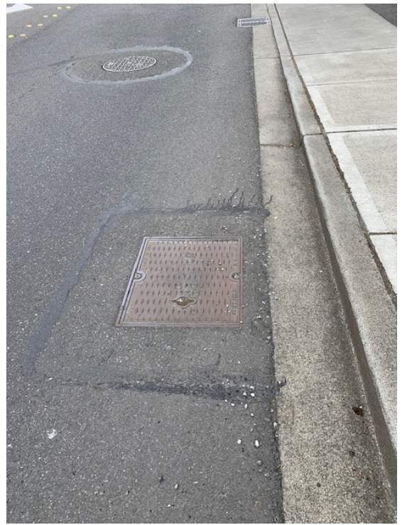
Catch Basin at Point P
