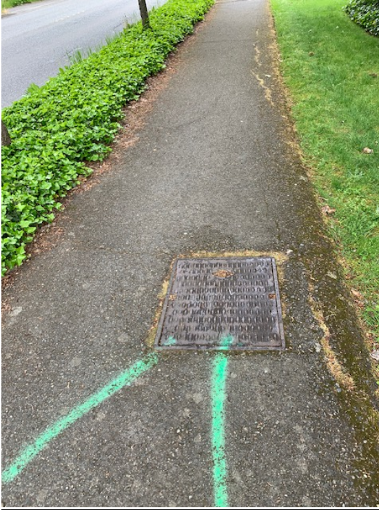
Catch Basin at Point M
