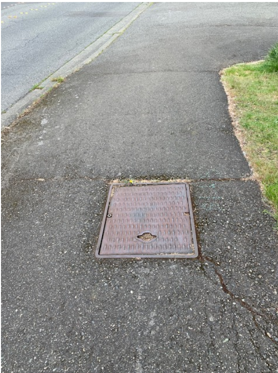
Catch Basin at Point N
