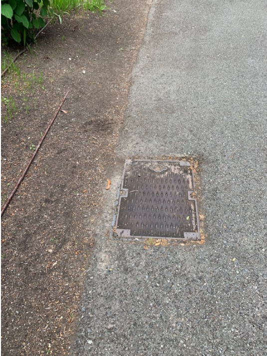
Catch Basin – At point B, Looking Downstream
