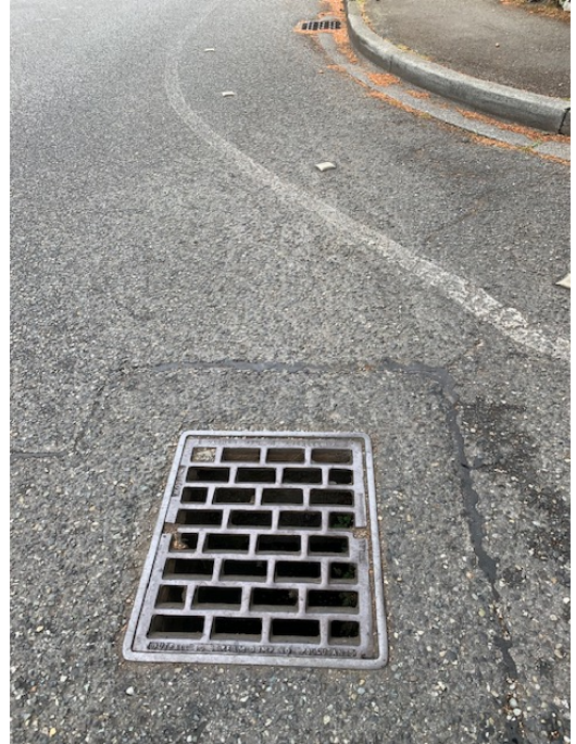
Looking Downstream from Catch Basin – At Point D
