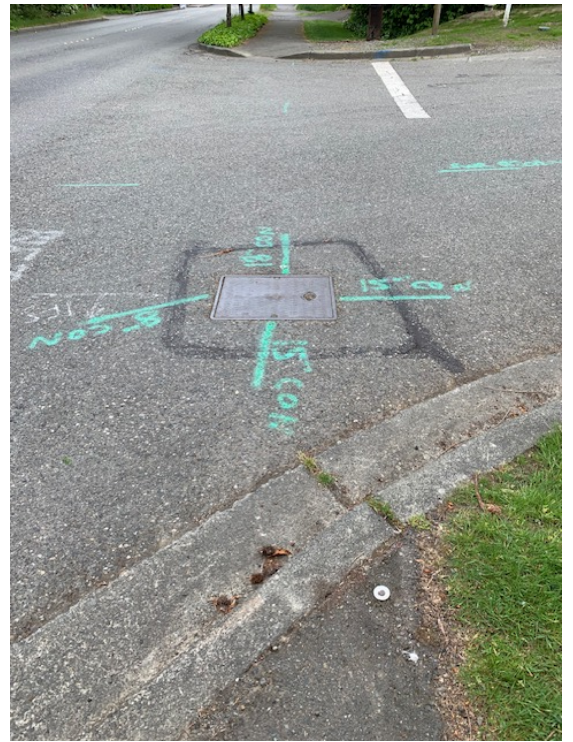
Catch Basin at point L
