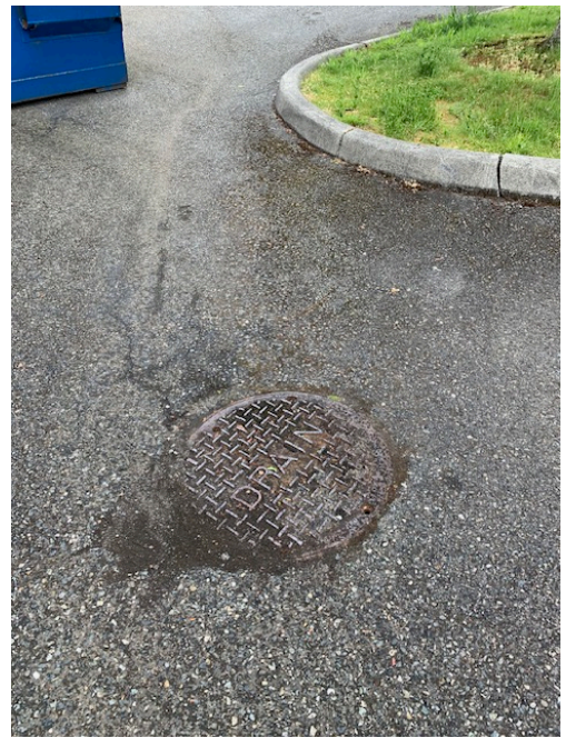
Catch Basin At Point T
