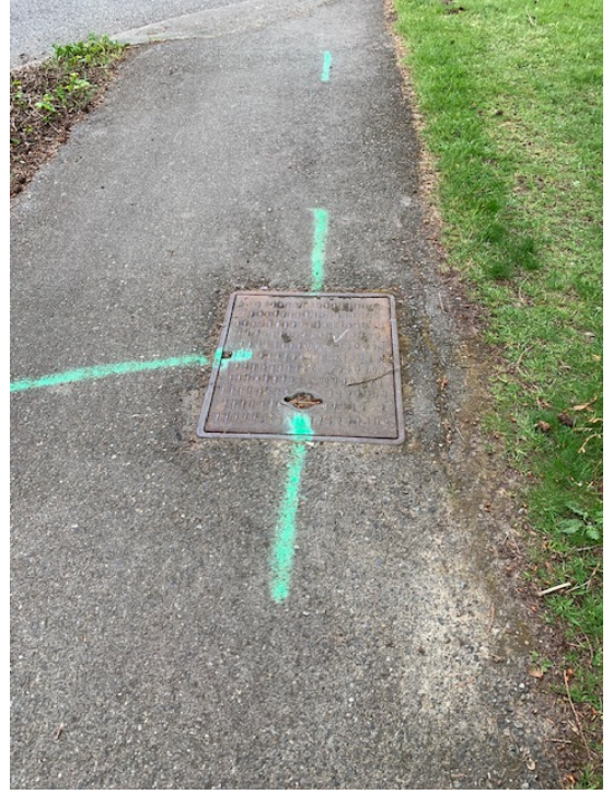
Catch Basin at Point K - Looking East
