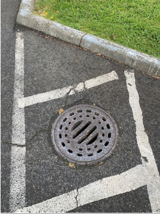
Catch Basin At Point U – Pipe water course
