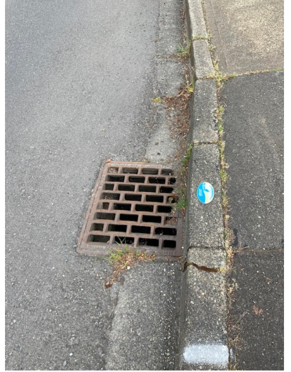
Catch Basin at Point O
