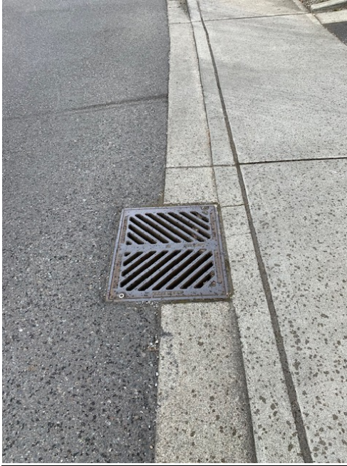
Catch Basin At Point Q at driveway
