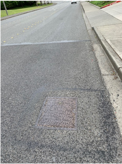
Catch Basin At Point R
