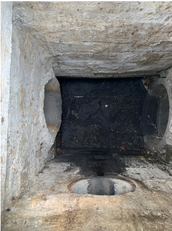
Inside Catch Basin – At Point B
